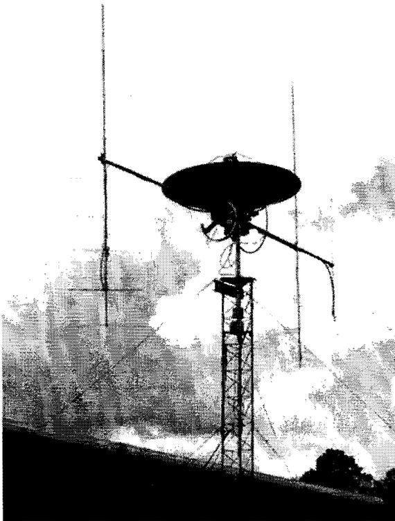
**Figure 4: S-Band and VHF Antenna Structure**
